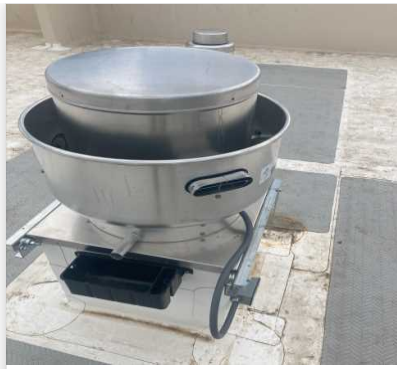
grease_cups_installed...
