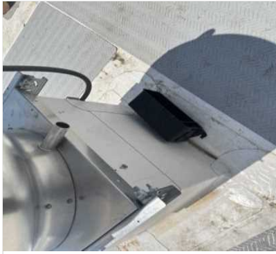
grease_cup_not_installed.jpe g
