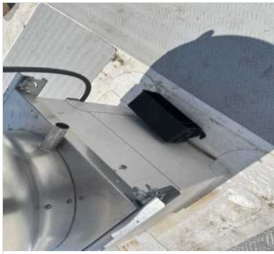
grease_cup_not_instal...
