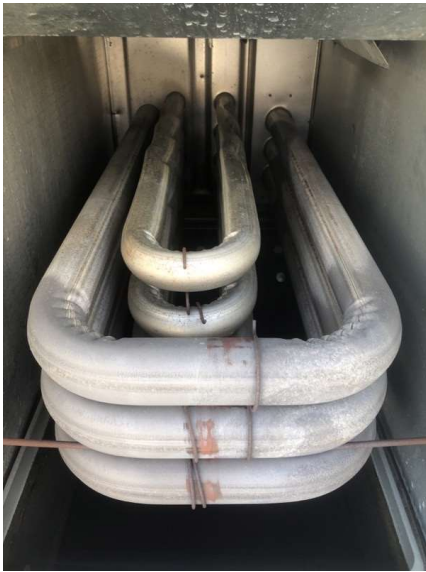
RTU-2 Burner Tube inspection
