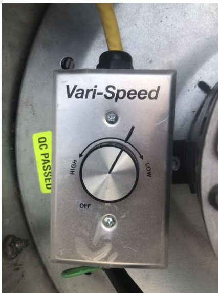
KEF-3 Fan Balanced, Setpoint marked
