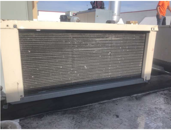
Walk-in Freezer Clean condenser
