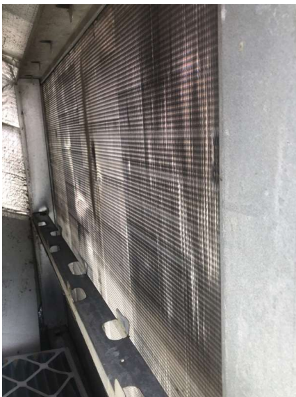
RTU-1 Clean evaporator coil
