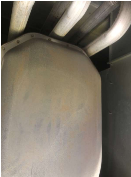
RTU-3 Burner tube inspection
