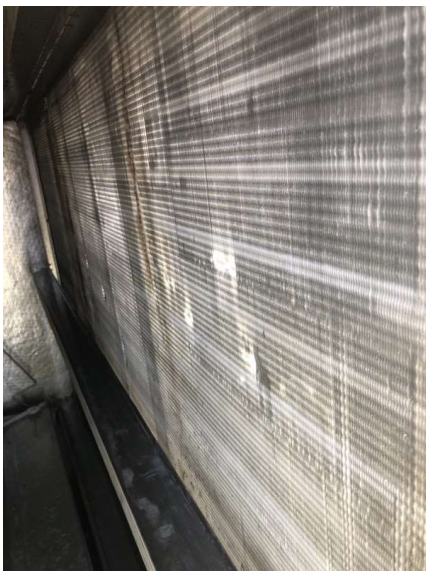
RTU-3 Clean evaporator coil
