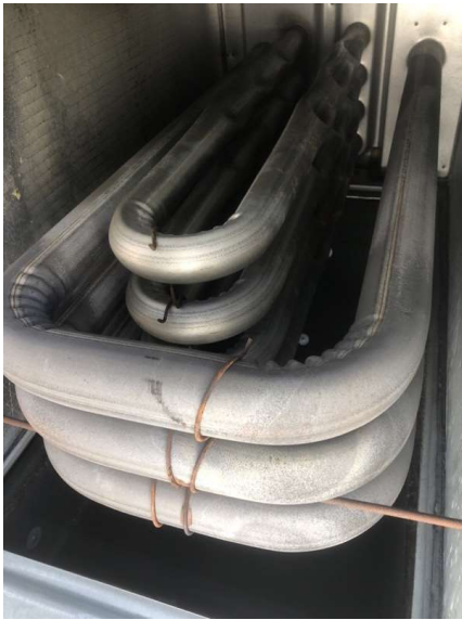
RTU-1 Burner Tube inspection
