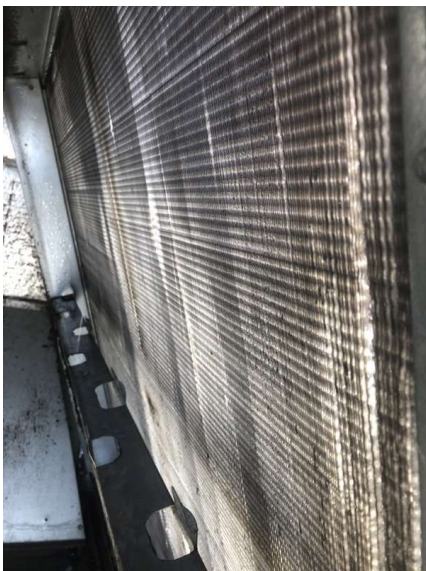
RTU-2 Clean evaporator coil
