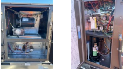
Interior Pictures of RTU Blower Section, Power / Control Section, Heat Section, Compressor Section.
