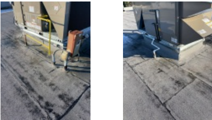
Roof Areas Around RTU Unit Showing the Areas are Clean and Free of Any Debris or Damage Related to the Installation.
