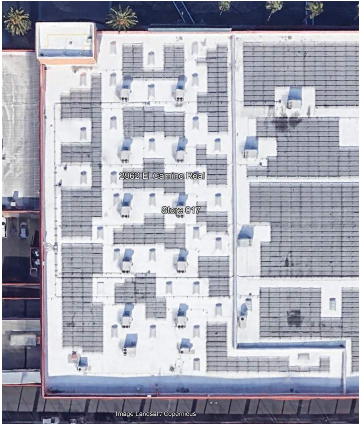
Photograph 1 – Aerial view of store via Google Maps
