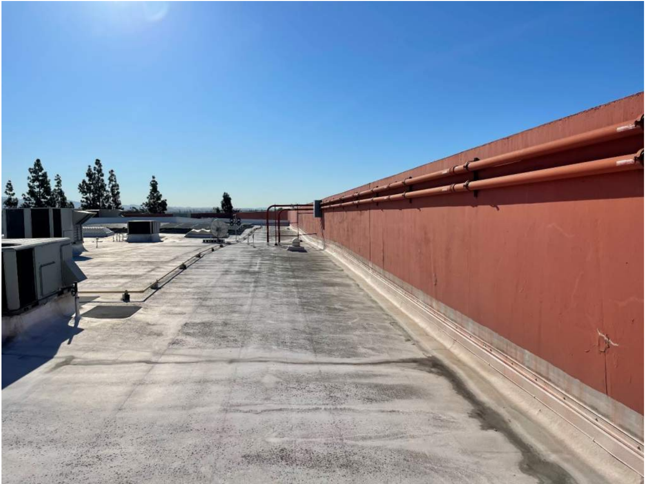
Photograph 7 – Overall photo of existing parapet wall
