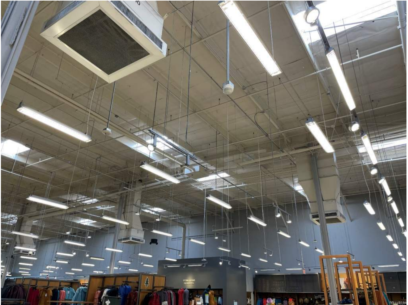
Photograph 3 – Overall view typical exposed structural framing
