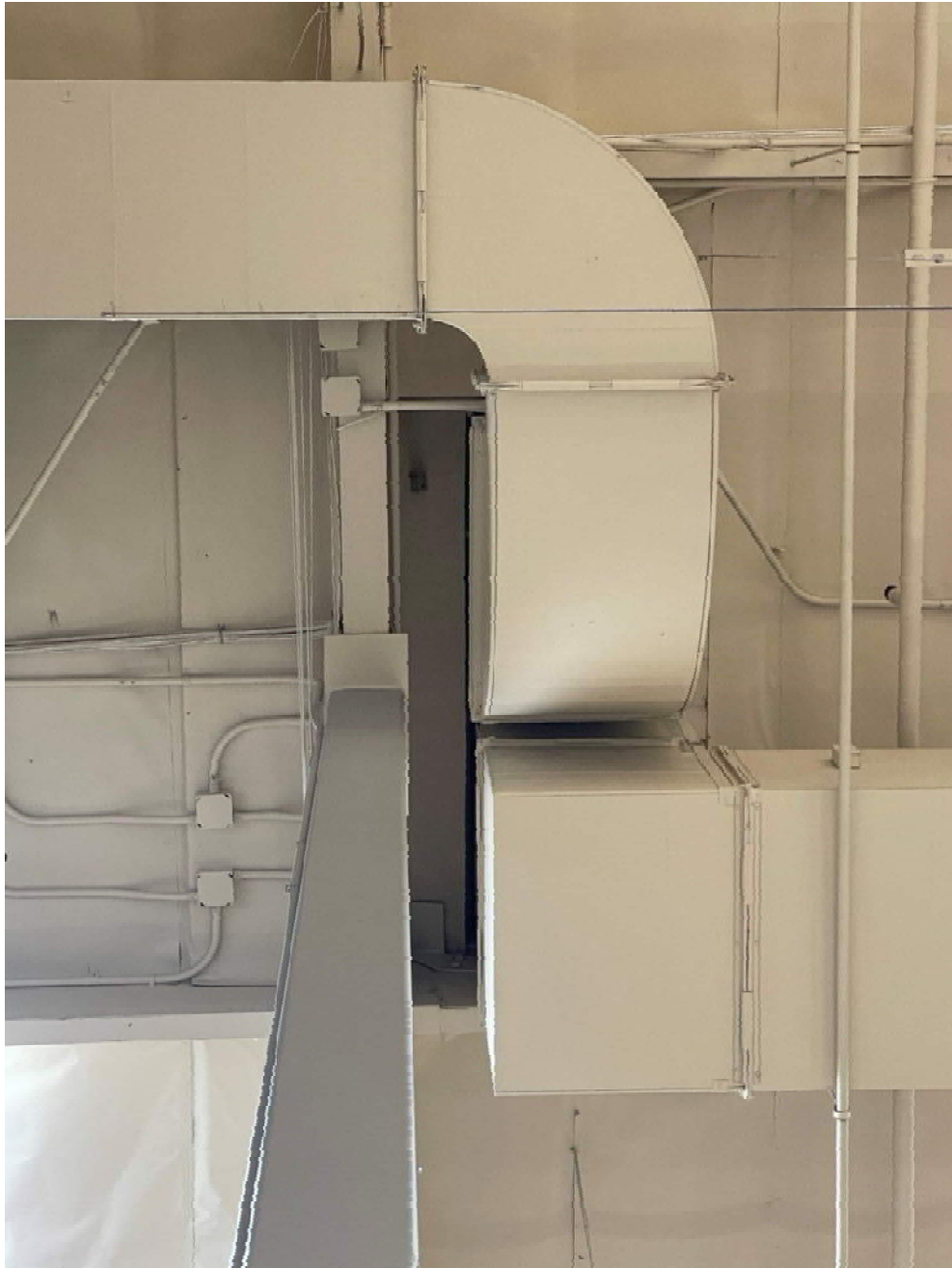
Photograph 5 – Overall view at underside of typical RTU
