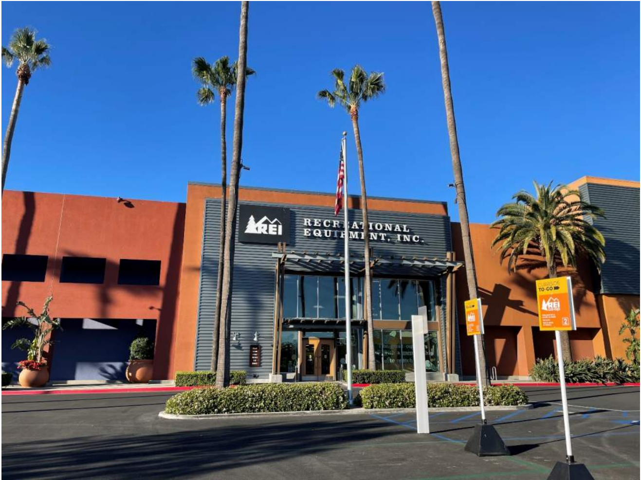
Photograph 2 – Overall view of store from parking lot
