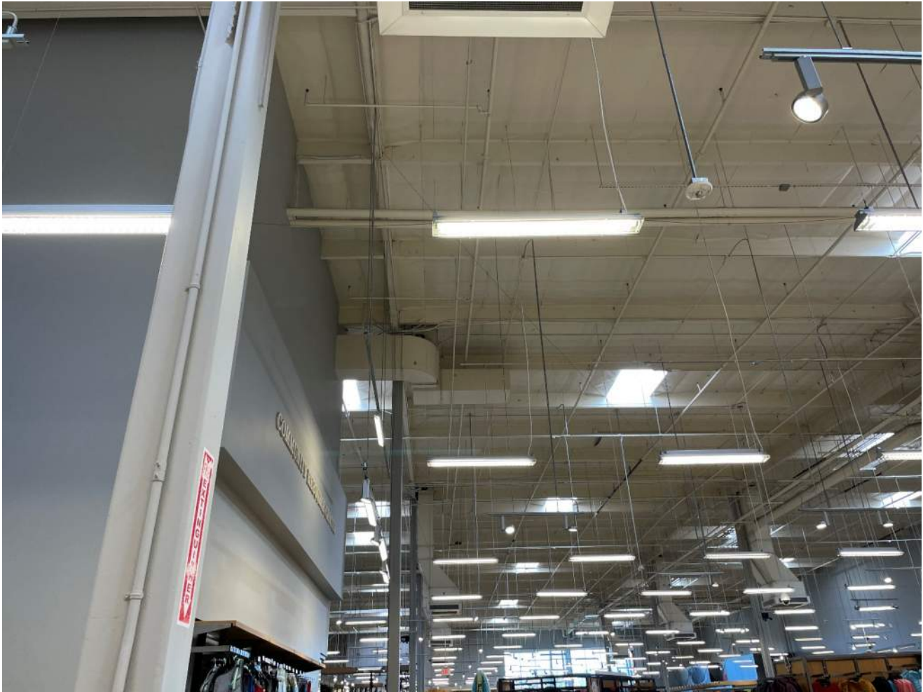
Photograph 4 – Overall view typical exposed structural framing
