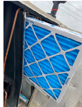
RTU-2 (KITCHEN) CLEAN EVAPORATOR FILTERS
