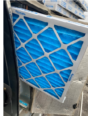
RTU-2 (KITCHEN) CLEAN EVAPORATOR FILTERS
