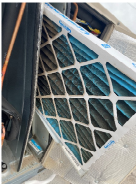
RTU-2 (KITCHEN) DIRTY EVAPORATOR FILTERS
