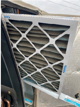
RTU-2 (KITCHEN) DIRTY EVAPORATOR FILTERS
