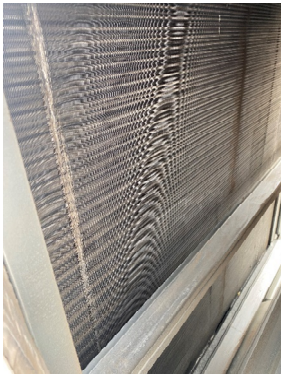
RTU-2 (KITCHEN) DIRTY EVAPORATOR
