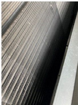
RTU-2 (KITCHEN) DIRTY EVAPORATOR
