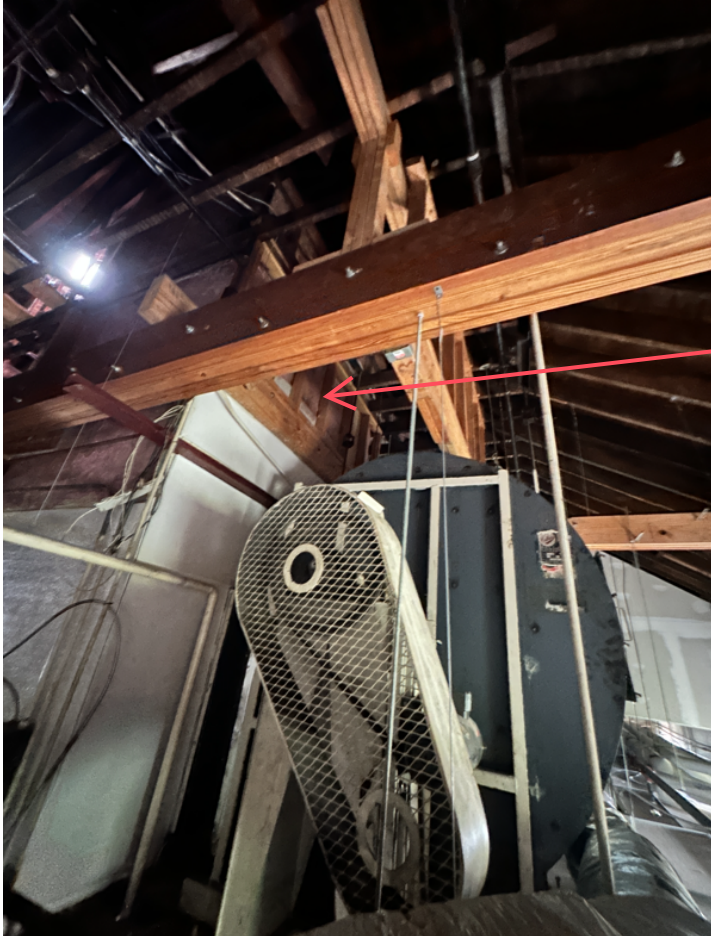
chimney out building.
