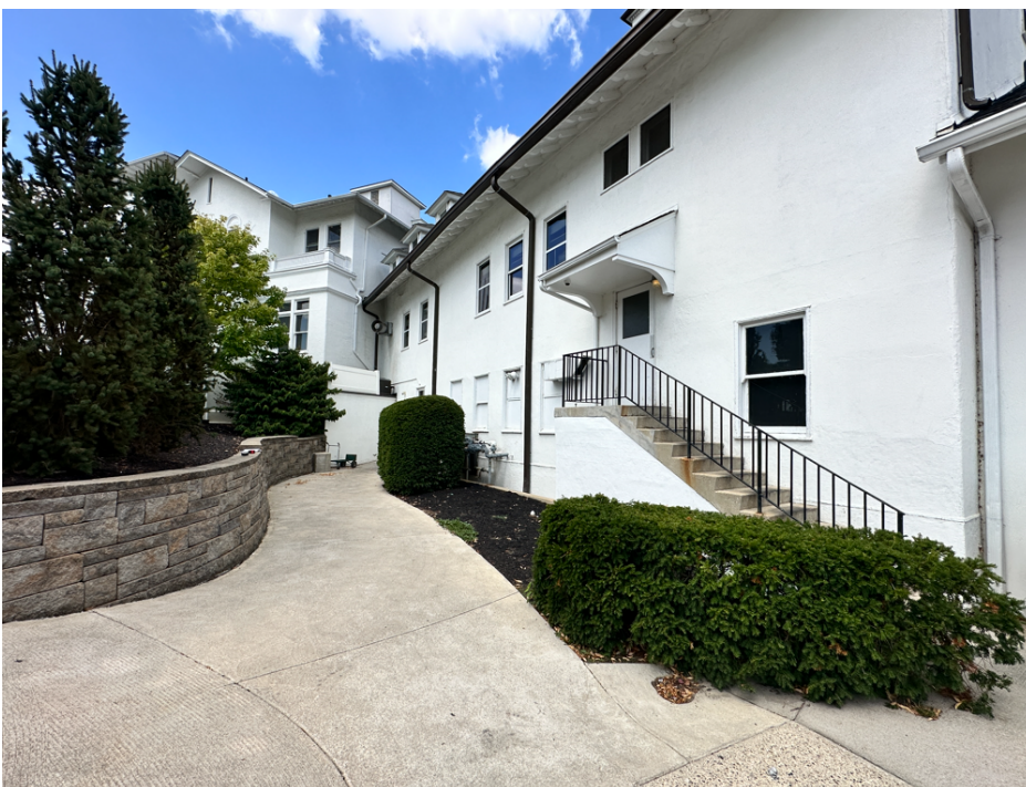
Lower service area out front. drawing sent previously with dimensional data of possible area for future MEP Assets.
