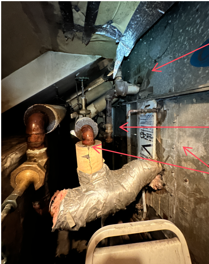
Supply blower behind CW Module
