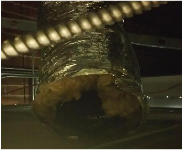
FLEX HANGING IN PHARMACY AREA WHERE VAV DIFFUSER GOES (CONSULTING)
