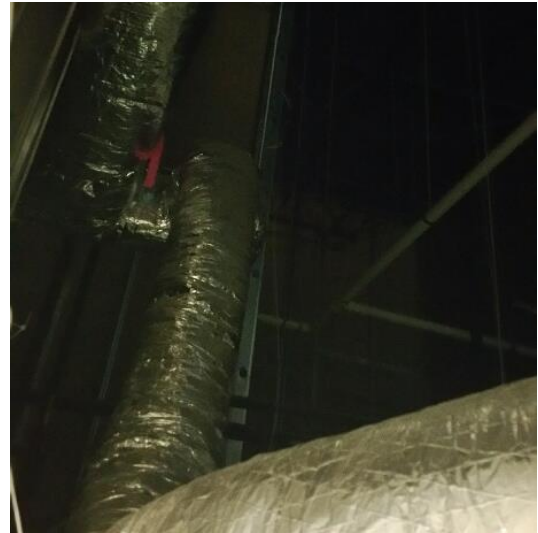
EXCESS AMOUNT OF FLEX IN PHARMACY AREA (REGISTER IN FRONT OF RESTROOMS)
