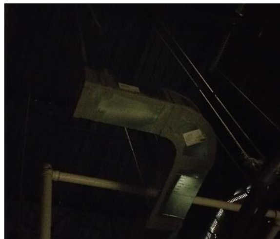
CAPPED OFF EXHAUST DUCTWORK IN THE LITTLE CLINIC AREA
