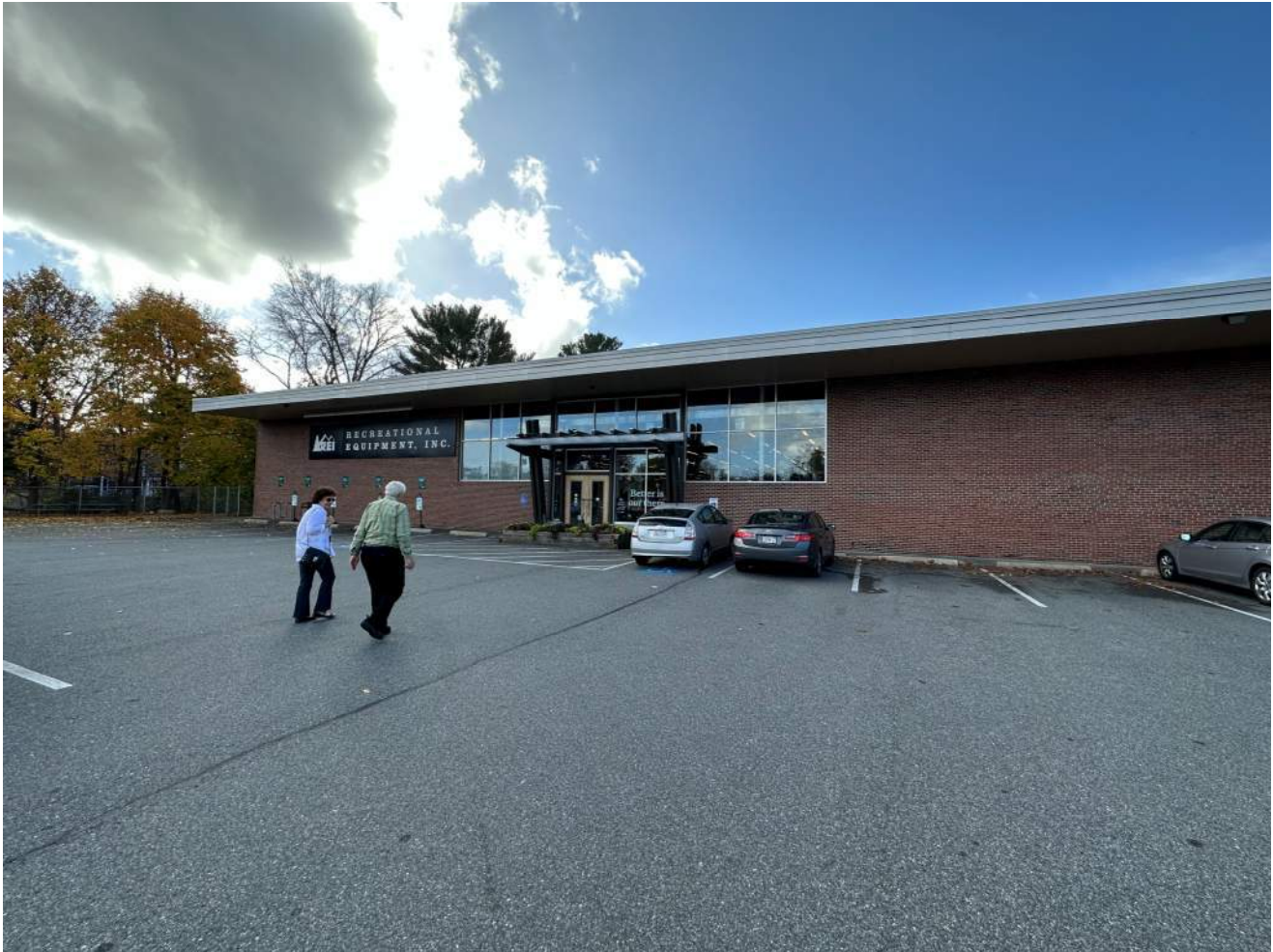
Photograph 2 – Overall view storefront entrance from parking lot
