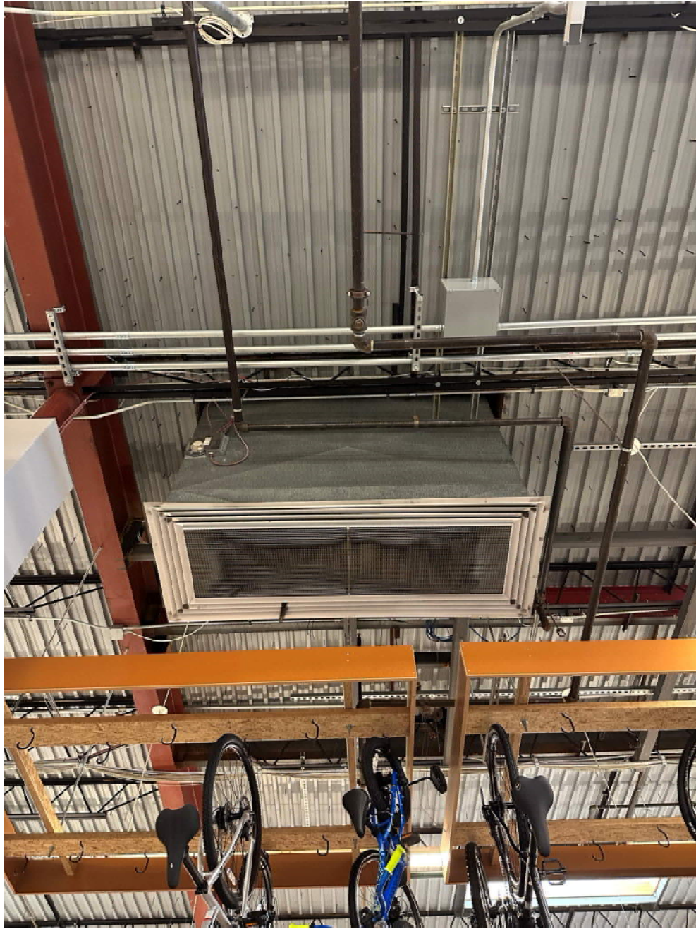
Photograph 5 – Overall view at underside of typical RTU 1-6
