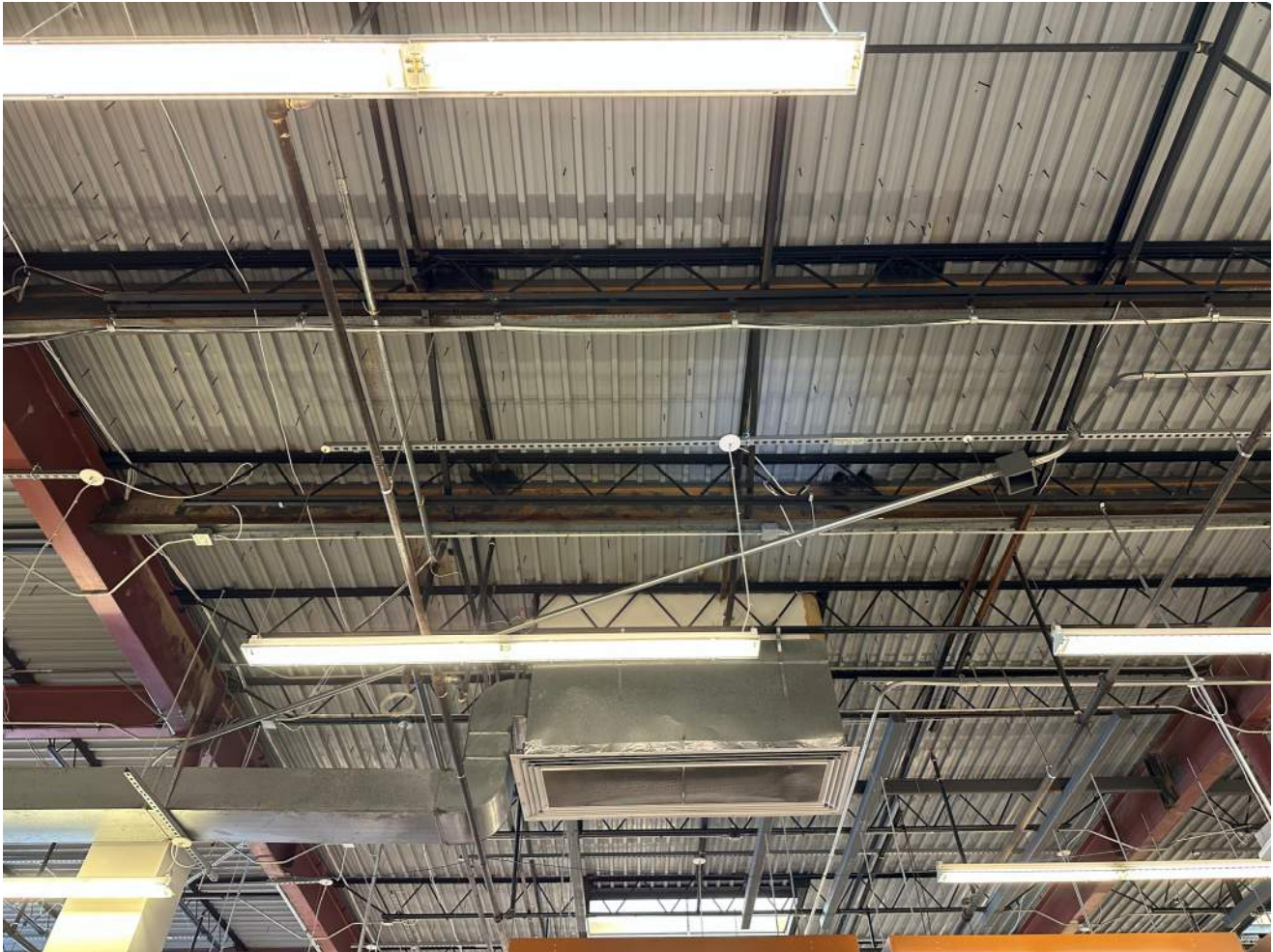
Photograph 4 – Overall view of typical exposed structural framing and W14x22 at RTU 1-6
