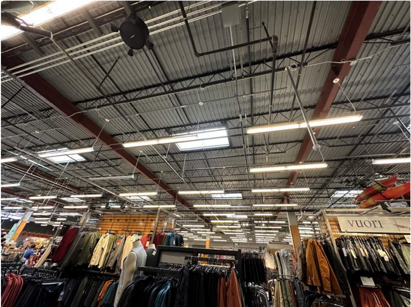
Photograph 3 – Overall view of typical exposed structural framing
