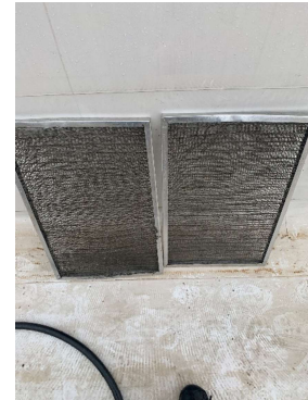
RTU-2 (KITCHEN) CLEAN OUTSIDE AIR FILTERS
