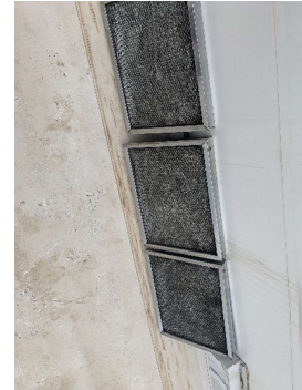
RTU-1 (DINING) CLEAN OUTSIDE AIR FILTERS
