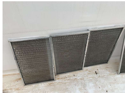
RTU-2 (KITCHEN) CLEAN OUTSIDE AIR FILTERS
