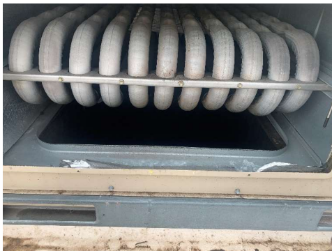
RTU-1 (DINING) BURNER TUBE INSPECTION
