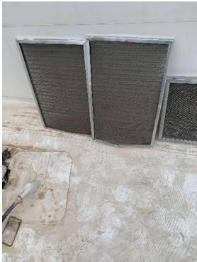
RTU-2 (KITCHEN) DIRTY OUTSIDE AIR FILTERS
