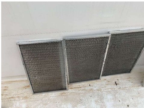
RTU-2 (KITCHEN) DIRTY OUTSIDE AIR FILTERS
