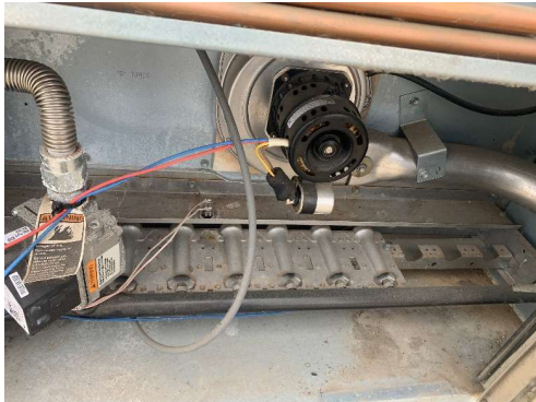
RTU-1 (DINING) BURNER TUBE INSPECTION
