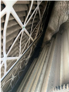
RTU-2 (KITCHEN) DIRTY EVAPORATOR FILTERS
