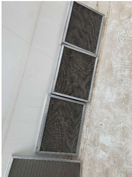
RTU-1 (DINING) DIRTY OUTSIDE AIR FILTERS
