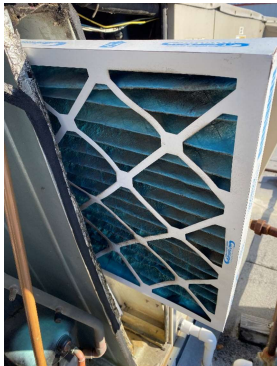
RTU-3 (DINING/RR) DIRTY EVAPORATOR FILTERS
