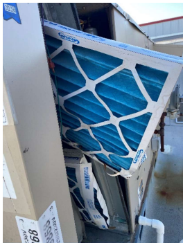
RTU-3 (DINING/RR) DIRTY EVAPORATOR FILTERS
