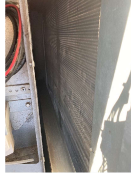
RTU-2 (FRONT KITCHEN/DINING) CLEAN EVAPORATOR
