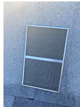
RTU-2 (FRONT KITCHEN/DINING) CLEAN OUTSIDE AIR FILTERS
