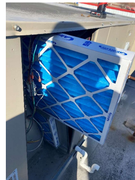
RTU-1 (DINING) CLEAN EVAPORATOR FILTERS
