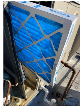
RTU-3 (DINING/RR) CLEAN EVAPORATOR FILTERS
