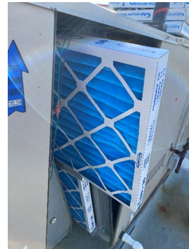
RTU-3 (DINING/RR) CLEAN EVAPORATOR FILTERS
