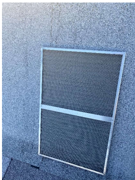
RTU-2 (FRONT KITCHEN/DINING) DIRTY OUTSIDE AIR FILTERS
