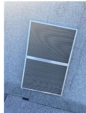
RTU-2 (FRONT KITCHEN/DINING) CLEAN OUTSIDE AIR FILTERS
