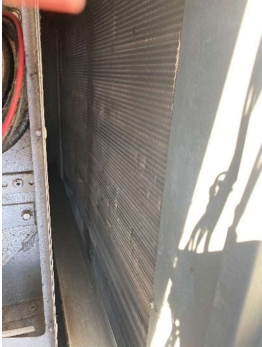
RTU-2 (FRONT KITCHEN/DINING) DIRTY EVAPORATOR
