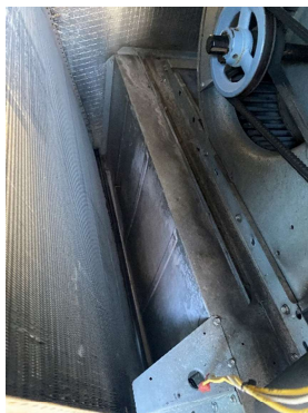
RTU-3 (KITCHEN) DRAIN PAN
