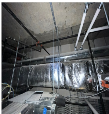
ISOLATORS_MISSING.jpeg
