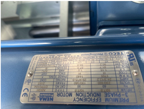
RTU-2 Motor nameplate
